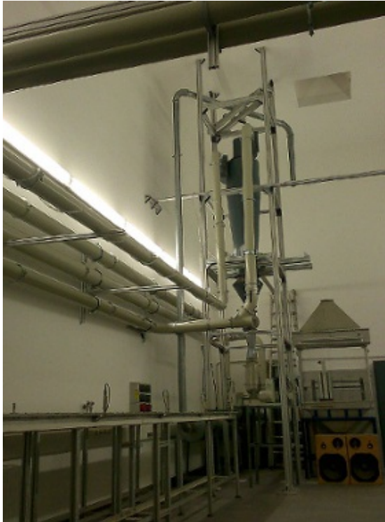
Flat channel for the experimental investigation of pneumatic conveying
